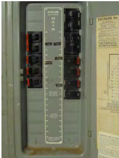
Typical electrical load center equipped with 'Stab-Lok' breakers by Federal Pacific
