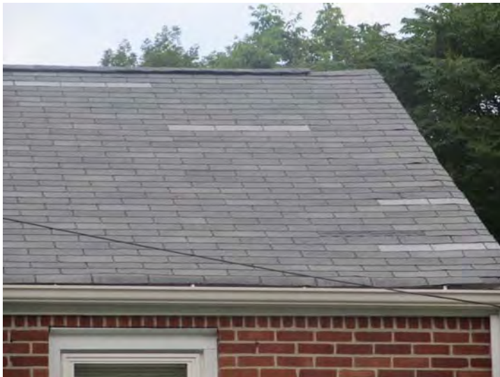
Older three-tab shingle roof coverings that exhibit age, wear, and past repair efforts are typical
