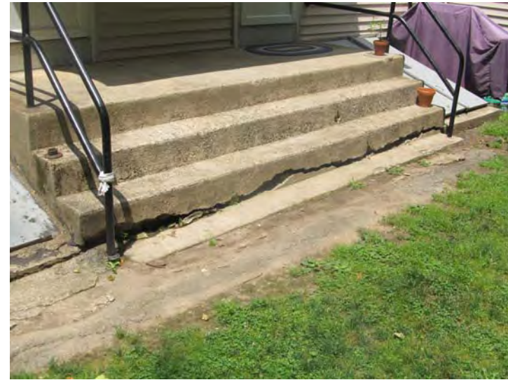
Concrete steps/stoops at unit entries exhibit varying levels of wear and deterioration
