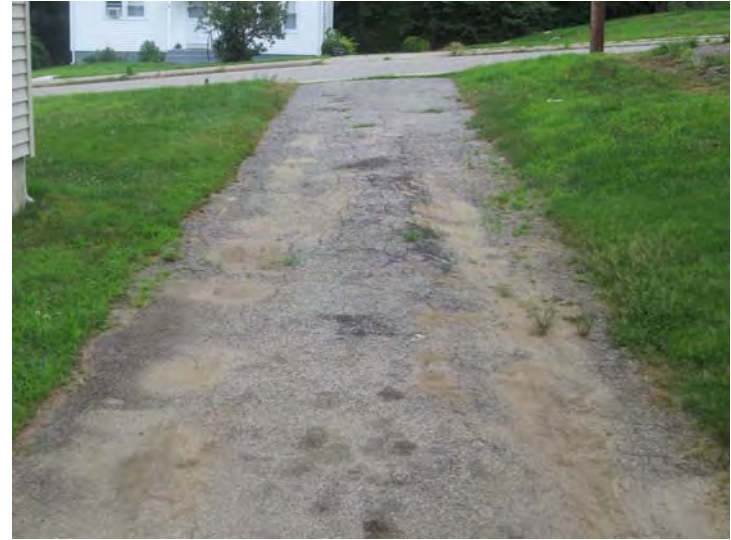
Typical condition of asphalt-paved driveway surfaces – Some replacement work recently completed
