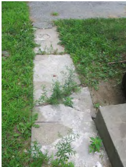
Secondary/interior sidewalks exhibit cracks and displacement at various locations
