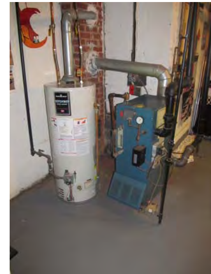
Each unit has a natural gas-fired steam boiler and domestic hot water tank
