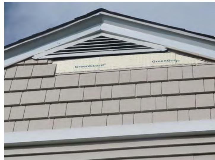
Isolated loose/missing pieces of vinyl siding noted
