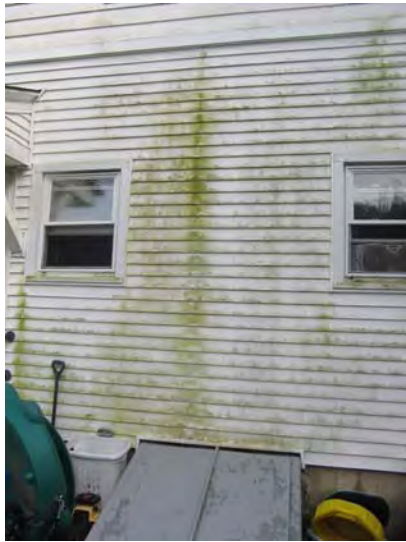
Dirt and organic growth on vinyl siding surfaces is widespread
